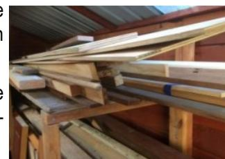
It is pretty easy to see how **stresses can be induced** in the timber on the right and it is surprising how quickly serviceable timber can be made unserviceable.
