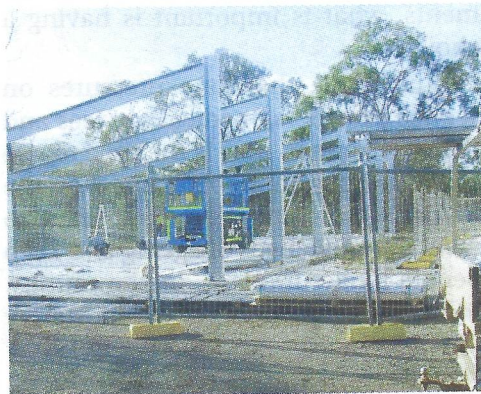
The skeleton of the shed.
