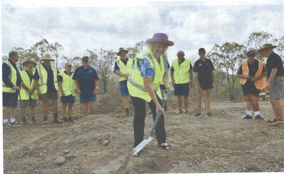
Desley Rail from Iwasaki Foundation turns the first sod.
